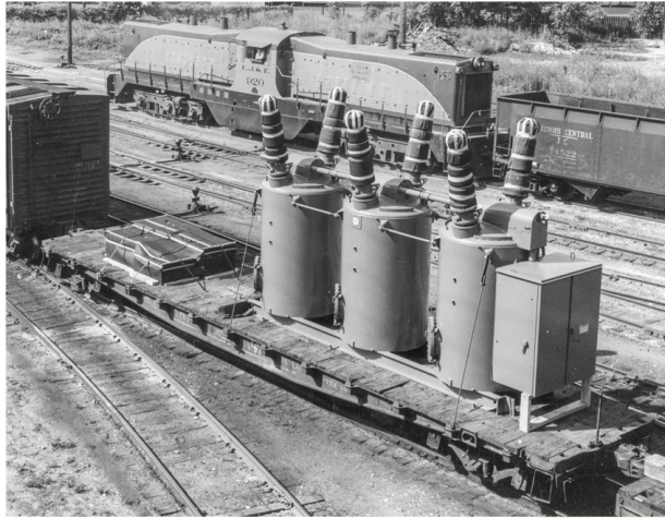
Joliet Illinois: 1958 Allis Chalmers BZO-HV oil circuit breaker load
