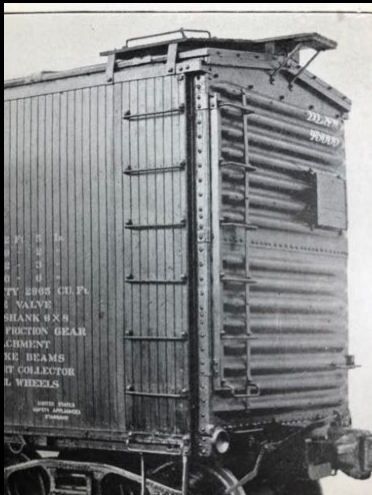
Grabs on side, grabs on angle and flat bar
